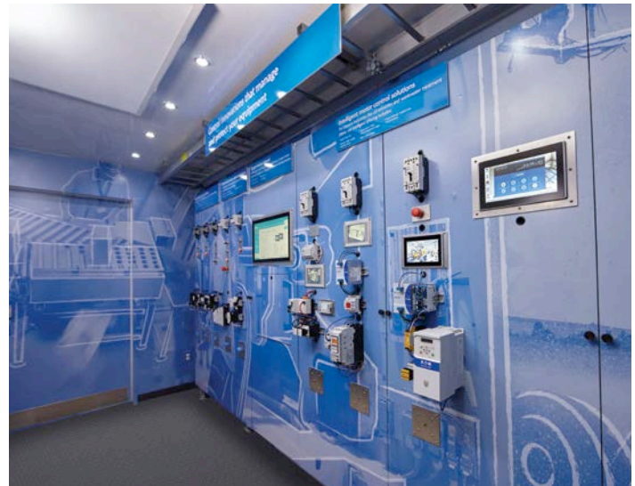
Full range of motor control capabilities, from basic to advanced to intelligent
